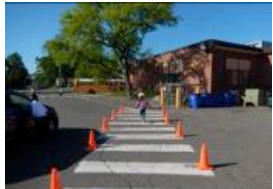
Figure 25: Faded Paint at crosswalk
