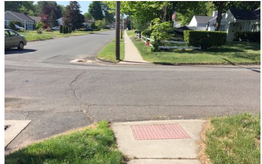
Figure 22: Missing Crosswalk across Dix Road to Southbound Mapleside Drive
