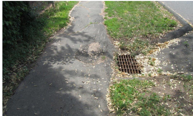
Figure 22: Deterioration of Pavement Condition along School Walk/Bike Path
