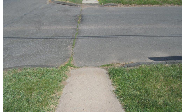
Figure 15: Longitudinal and Transverse Cracking at Wolcott Hill Road and Cumberland Avenue
