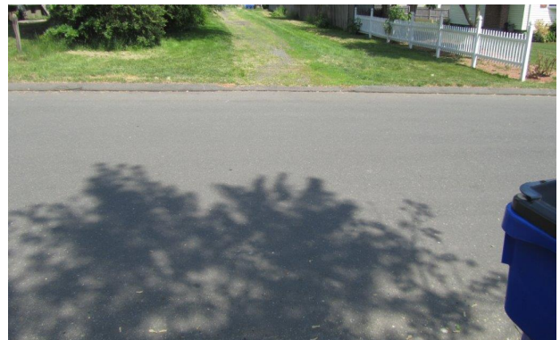
Figure 26: Lack of Crosswalk or Curb Ramps for Crossing Oxford Street from Gravel Path
