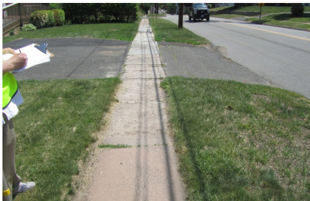
Figure 13: Sidewalk along Nott Street in Poor Condition
