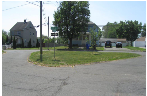
Figure 19: Longitudinal and Transverse Cracking at Cumberland Avenue and Buckland Road
