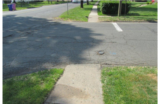
Figure 8: Poor Pavement Condition at Wolcott Hill Road and Robbins Drive
