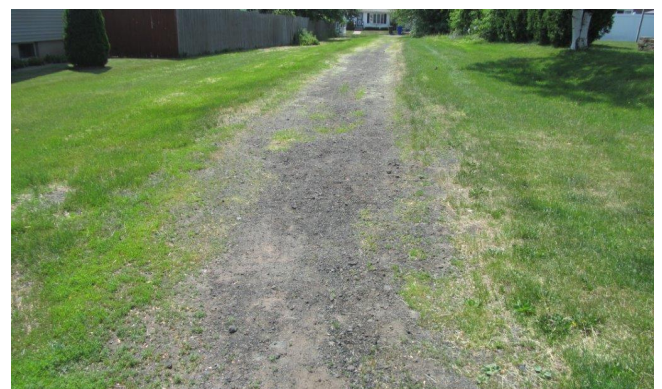
Figure 21: Poor Surface Condition on Gravel Path
