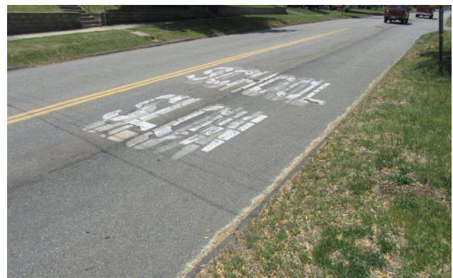
Figure 9: Poorly Painted SCHOOL SLOW Pavement Markings
