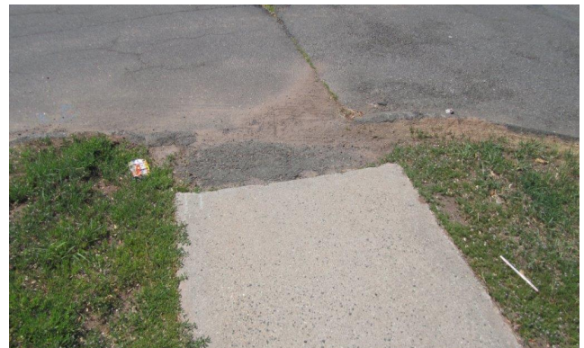
Figure 17: Poor Condition of Curb Ramps at Wolcott Hill Road at Cumberland Avenue
