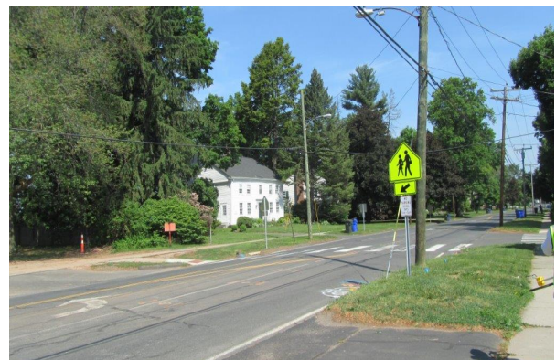
Figure 24: Newly Installed Signs Crowding Older Signs
