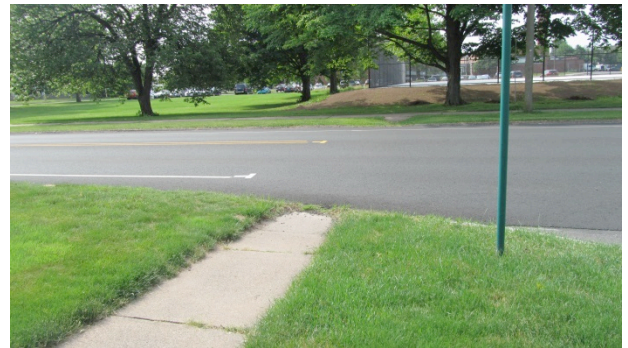
Figure 11: Handicap Ramp in Close Proximity to Wells Road/Willow Street Signalized Intersection
