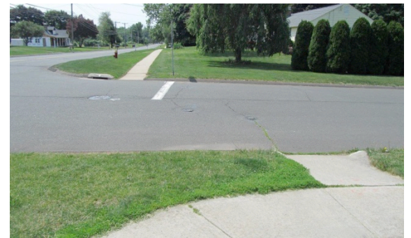
Figure 17: Offset Handicap Ramps at Nathaniel Drive
