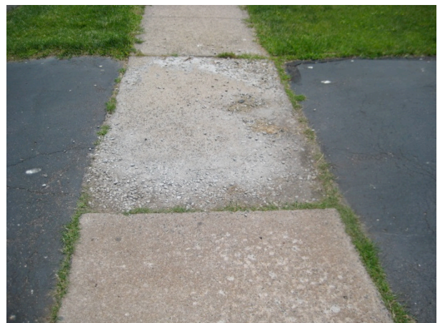
Figure 14: Broken Sidewalk through a driveway on Glenwood Drive
