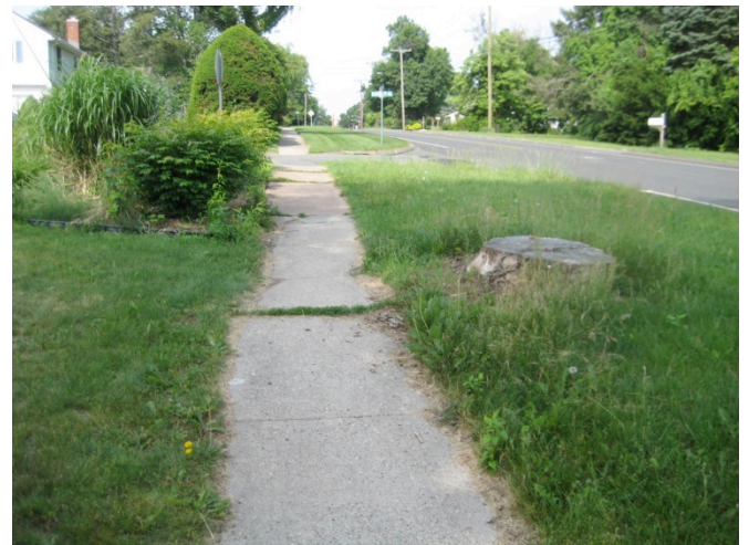
Figure 10: Upheaved sidewalk on Wells Rd West of Cedar St
